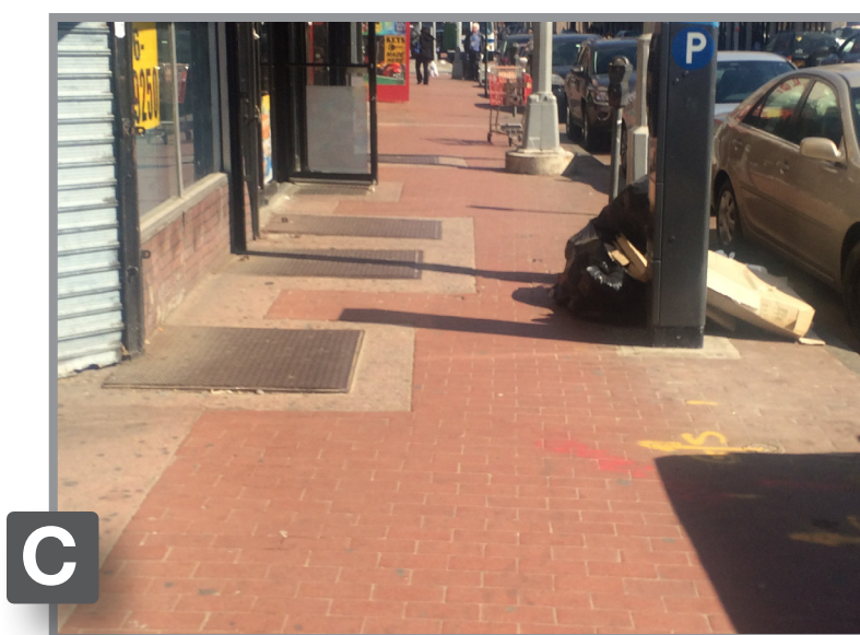
C Red brick pavers are the prominent sidewalk material. Retail basement access, vents, and vaults can be found between Sutphin Boulevard and 150th Street.
