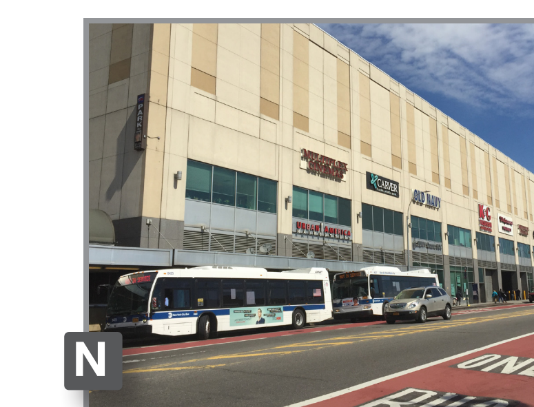
N ROW varies from 40 feet (at Sutphin Boulevard), to 72 feet (east of Parsons Boulevard). Bus lanes operate in both directions.
