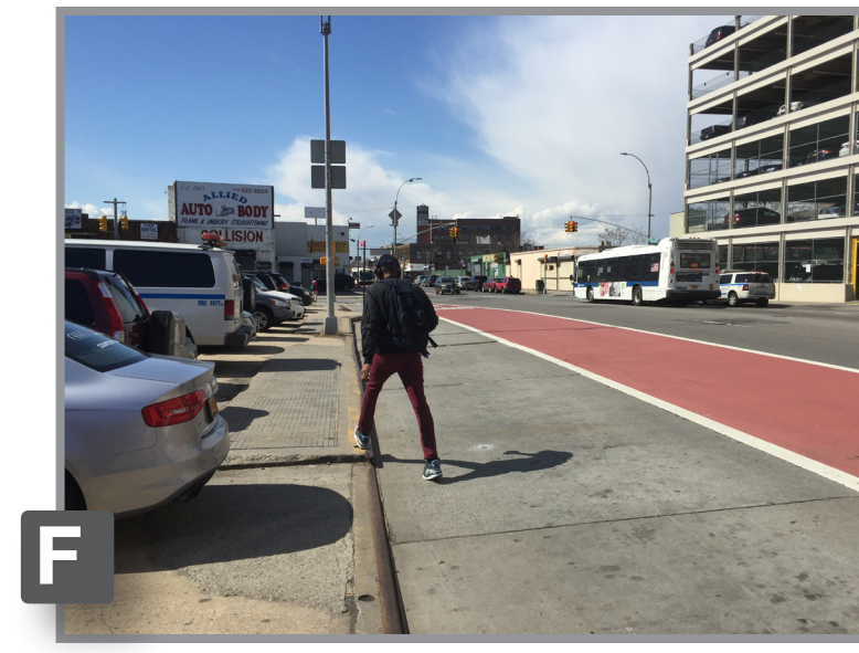
F Triangular site currently utilized for bus transfers with resulting awkward road operations and geometry. Unsafe for pedestrians.
