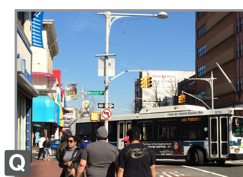
Q Overall lighting levels meet standards. Distinctive art deco style TBTA Poles used throughout corridor at approximately 75 foot spacing. No pedestrian scaled lighting.
