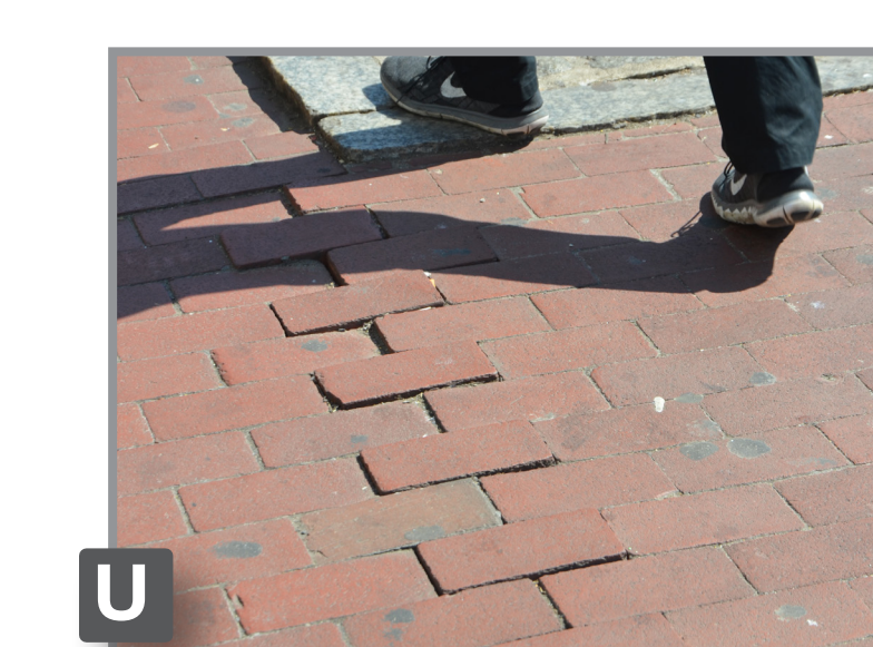
U Strong presence of red brick pavers from Sutphin Boulevard to 169th Street. Although a distinct feature, some bricks were observed to be dislodged.
