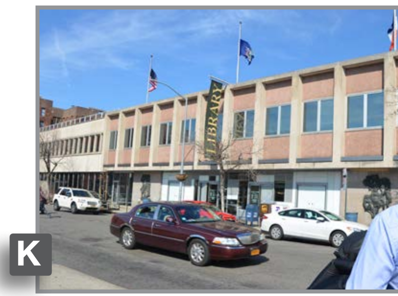
The Queens Library, a regional destination, is a synergy of the original Brutalist building and modern architectural styles.
