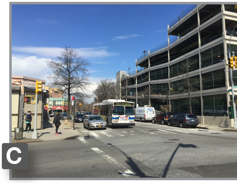
C Many parking garages along the corridor.
