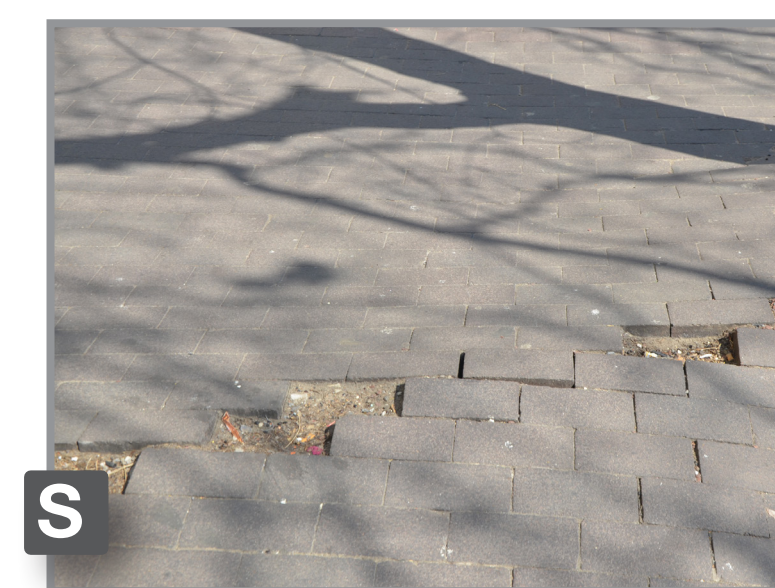
S Good to poor sidewalk conditions, with varying materials of concrete and brick pavers.
