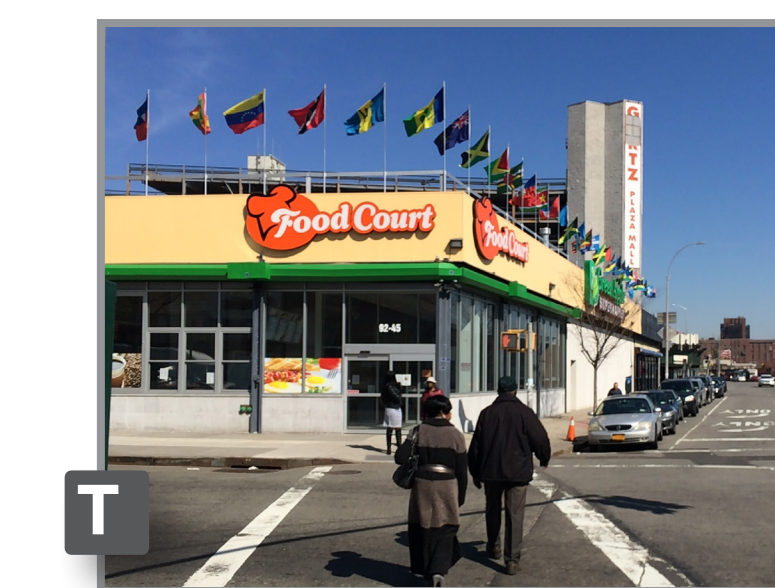
T Long pedestrian crossings at intersections with faded markings. Some T-intersections without pedestrian crossings.
