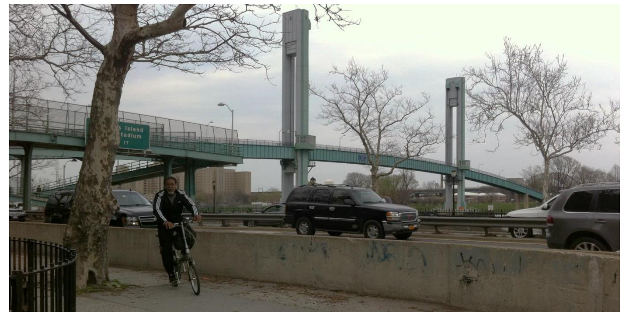
Existing: E 102 nd St Greenway access, facing north
