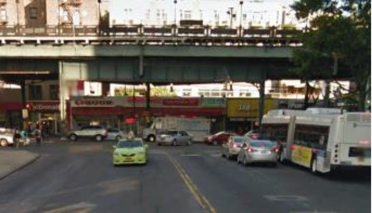
Existing: W 225 th St, Bronx facing west
