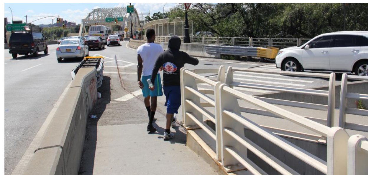
Existing: Macombs Dam Bridge, facing west
