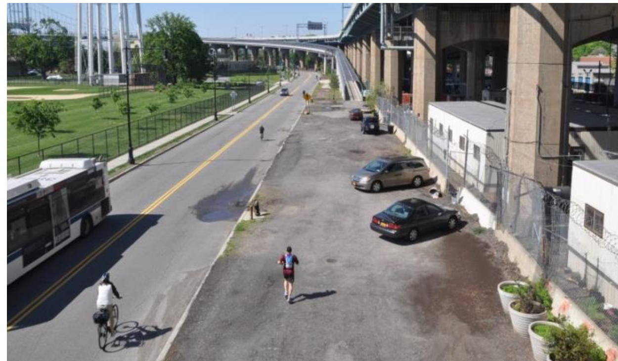
Existing: Hell Gate Cir, facing south
