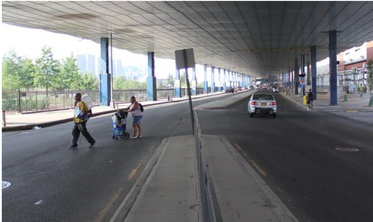
Existing: Gateway Center Blvd, facing northeast
