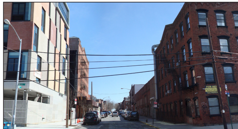
Modern residential development (left) across From 19th century brick factory (right) in Greenpoint, Brooklyn
