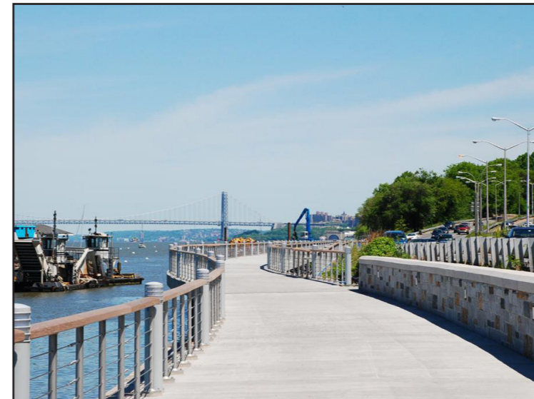
Multi-use path connection built on a pile-supported structure over the open water in Riverside Park, Manhattan
