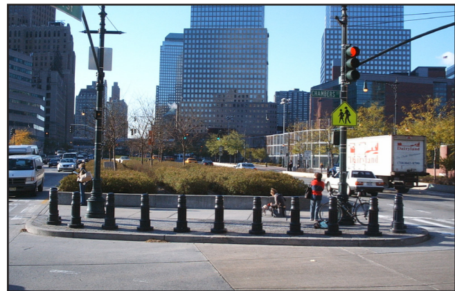
Pedestrian refuge with cast Iron bollards, Route 9A, Manhattan
