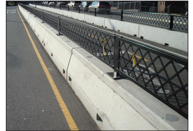
Reinforced concrete divider with railing, Sands Street, Brooklyn
