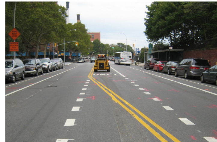
View north on Navy Street looking towards Sands Street (existing)
