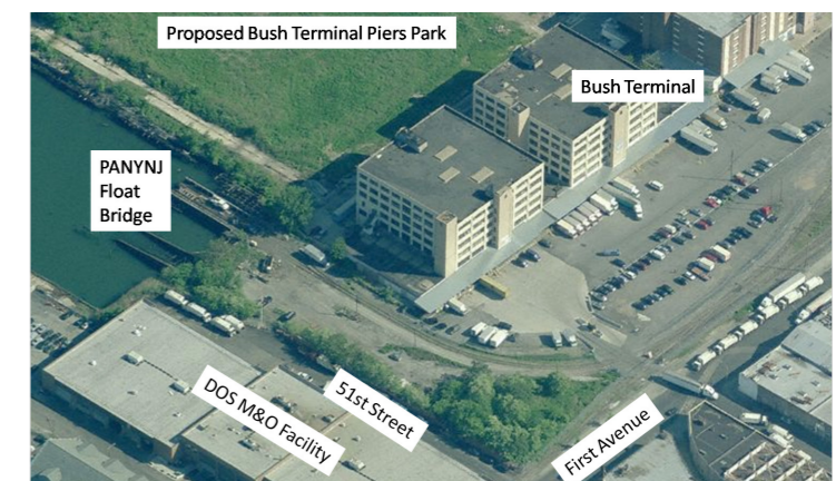
Float bridge operations at 51st Street (existing). Photo: Bing
