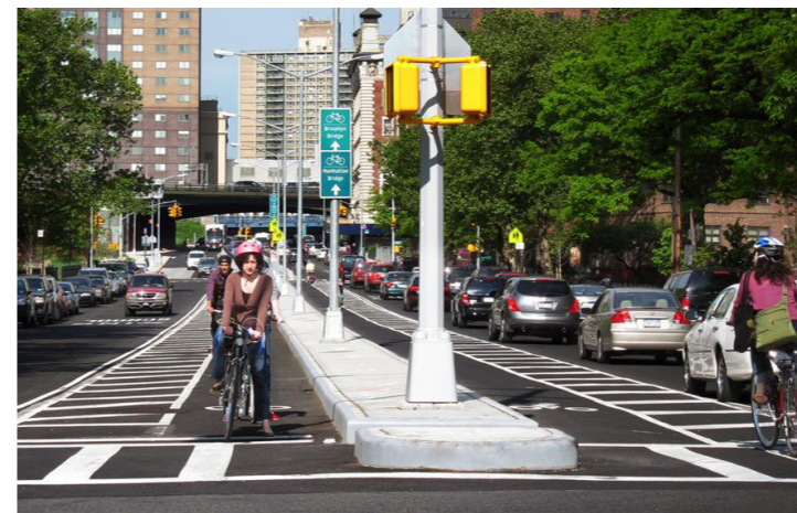
Grade-separated bicycle lane on Sand Street (existing)
