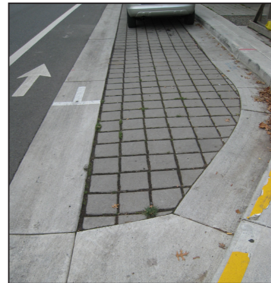
Porous pavers in parking lane
