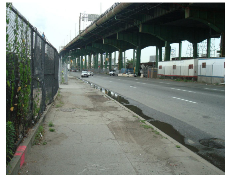
Hamilton Avenue looking west from Department of Sanitation Marine Transfer Station (existing)
