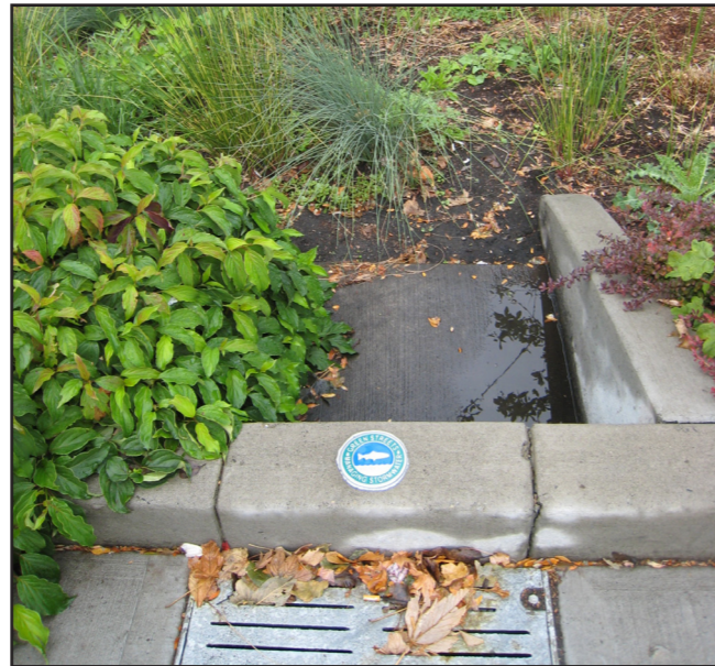
Storm drain outfall to rain garden, Portland, OR
