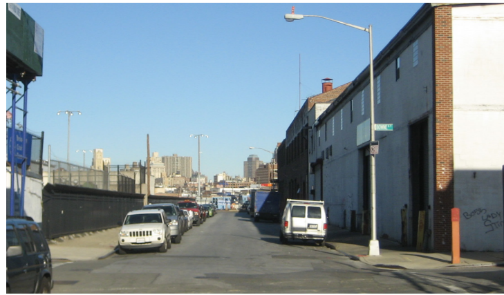
Imlay Street north of Bowne Street (existing)
