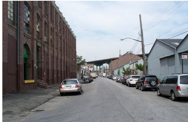
Smith Street between Sigourney Street and Bay Streets (existing)
