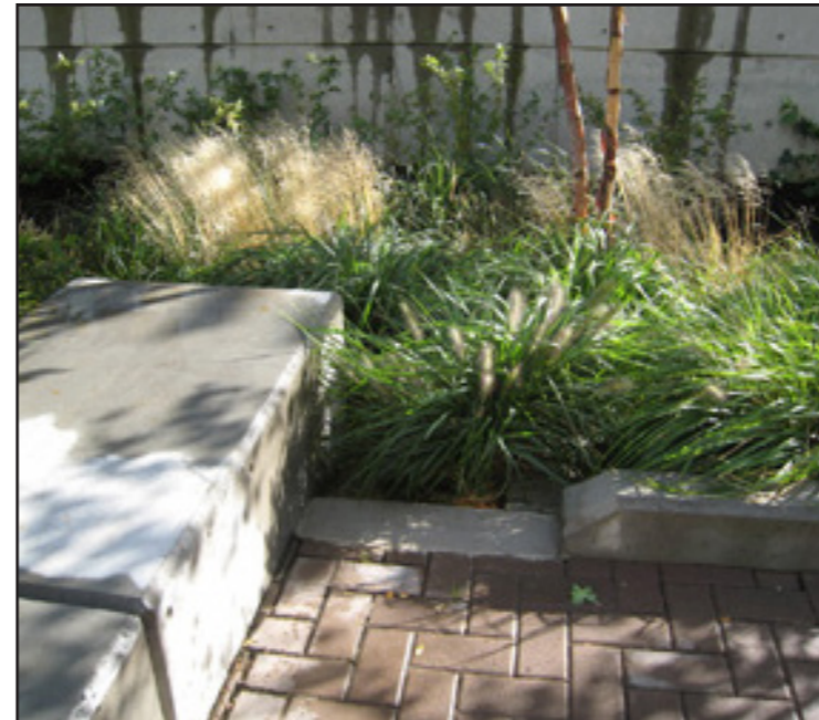
Slotted curb allows stormwater capture, Portland, OR
