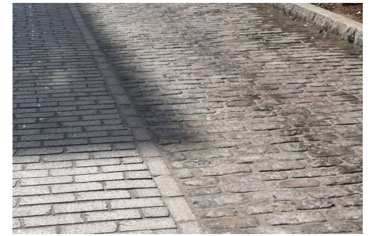
Smoothed cobblestone treatment on Washington Street, DUMBO (precedent for Plymouth/Water Street and Hudson Avenue)
