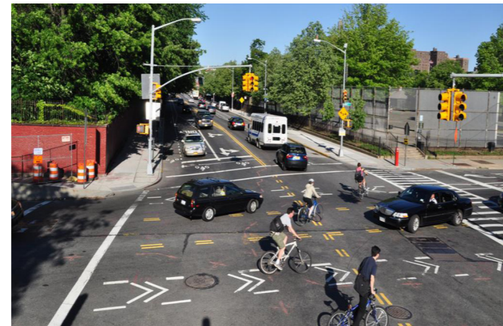
View looking east down Flushing Avenue from Navy Street (existing)
