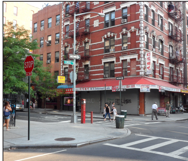
Curb extension implemented in conjunction with school crosswalks, Manhattan
