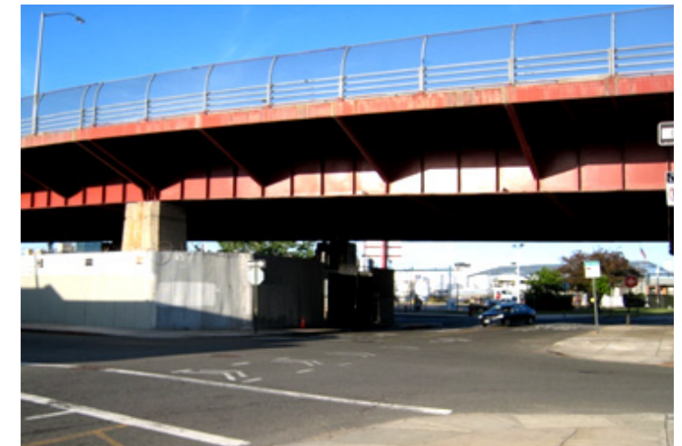
Box Street at the Pulaski Bridge (existing)
