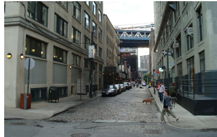
Plymouth Street looking west from Jay Street (existing)
