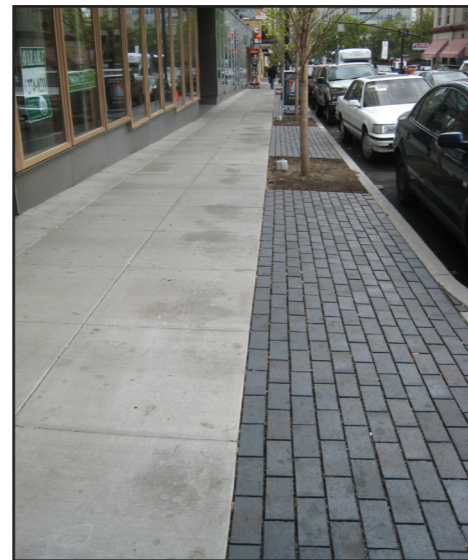
Porous pavers in amenity strip
