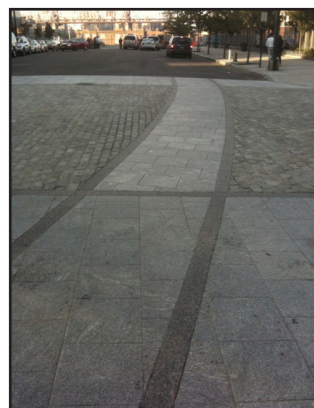
Stone and Belgium block patterns provide smooth surface for cyclists, Queens West
