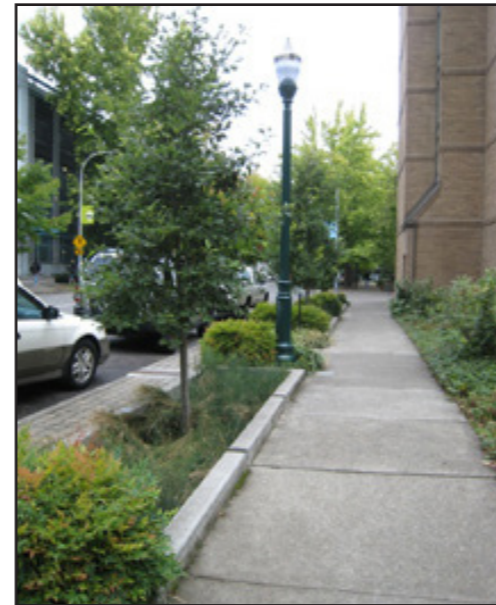
Slotted curb rain garden, Portland, OR
