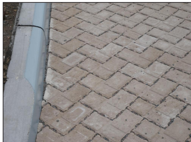
Porous pavers in parking lot, Brooklyn Navy Yard, Brooklyn
