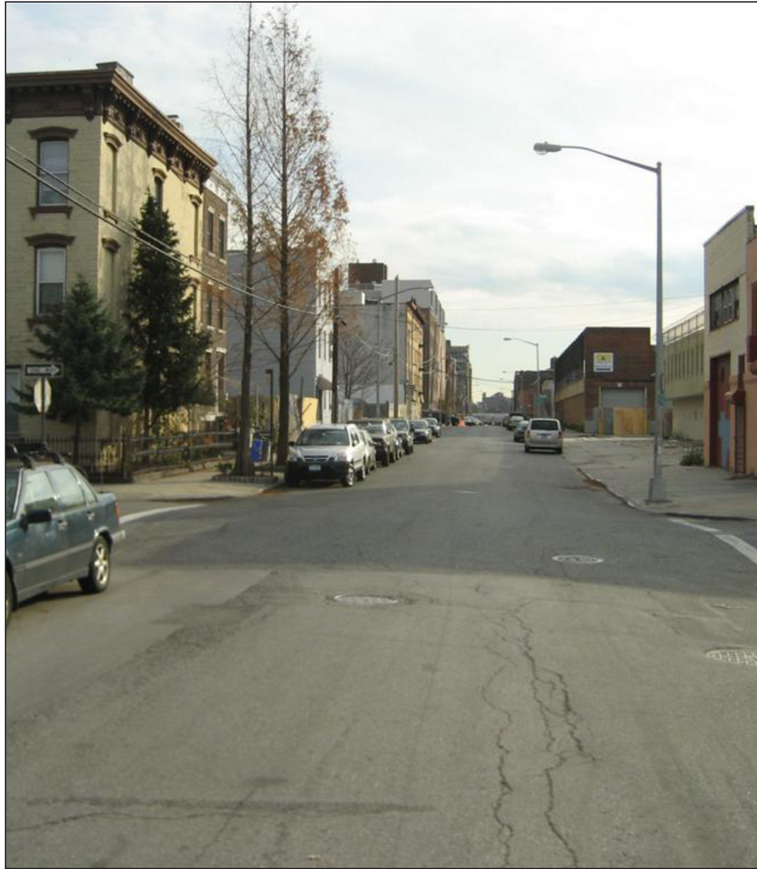
Existing conditions on West Street
