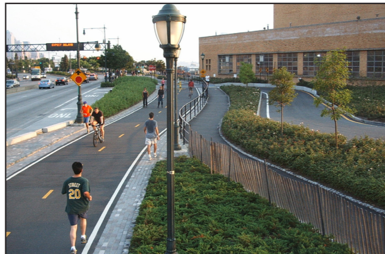
Off-street multi-use pathway with separation between bikes and pedestrians, Route 9A Bikeway/Walkway, Manhattan
