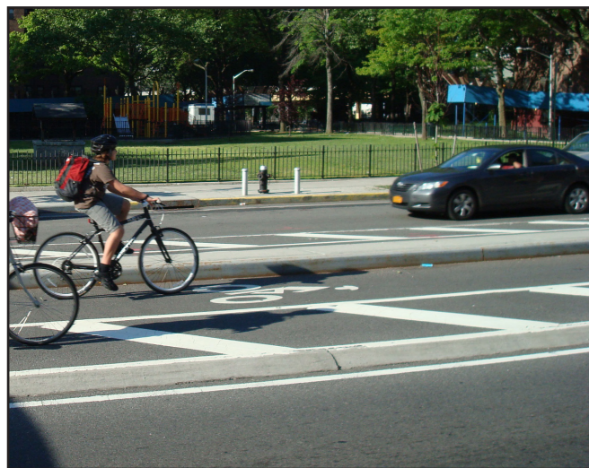
Grade-separated bicycle lanes alongside a raised median, Sands Street, Brooklyn
