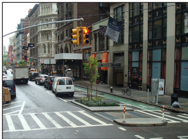
Pedestrian island with planting and flexible bollards, Manhattan
