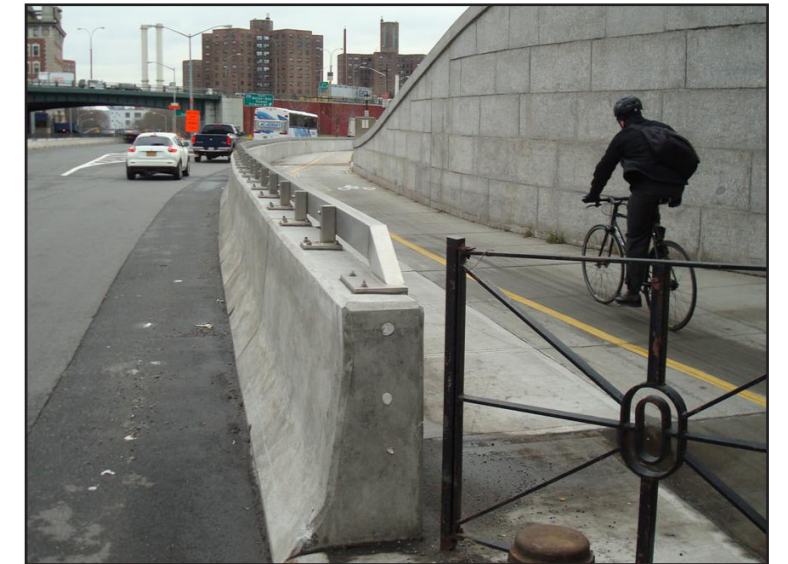
Reinforced concrete divider with railing, Manhattan Bridge Approach, Brooklyn
