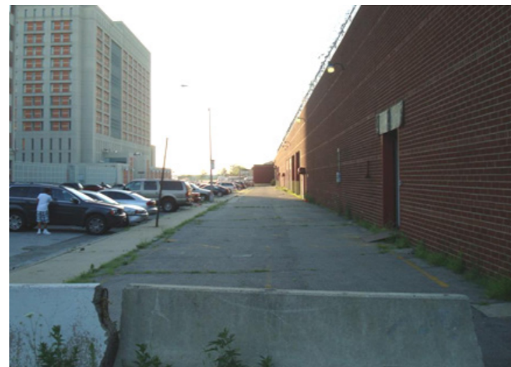
29th Street looking west from Third Avenue (existing)
