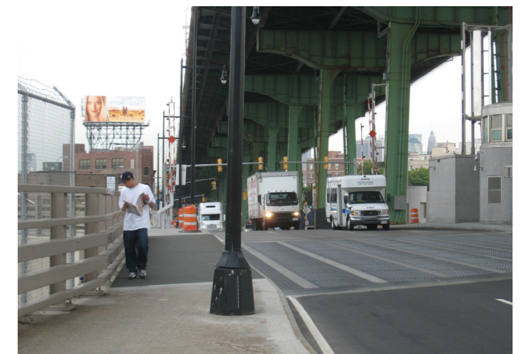
Hamilton Avenue Bridge over Gowanus Canal facing west (existing)
