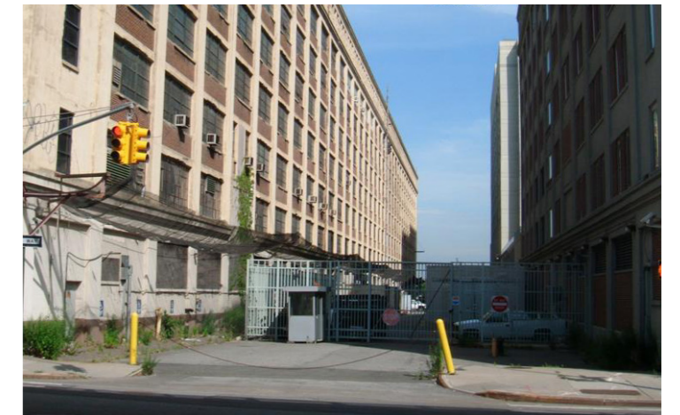
30th Street looking west from Third Avenue (existing)
