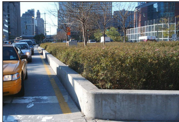
Planted roadway medians, Route 9A, Manhattan
