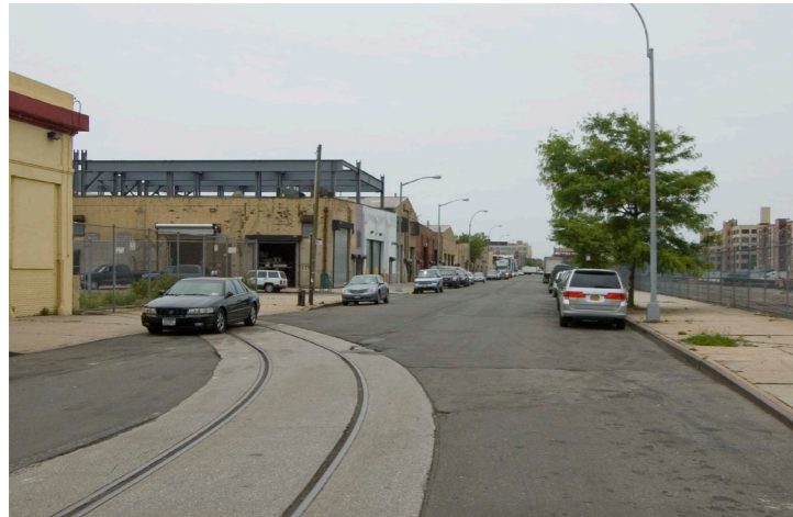
First Avenue facing south from 43rd Street (existing)
