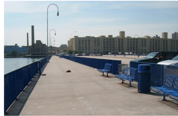
58th Street Pier view looking east with BAT in background (existing)
