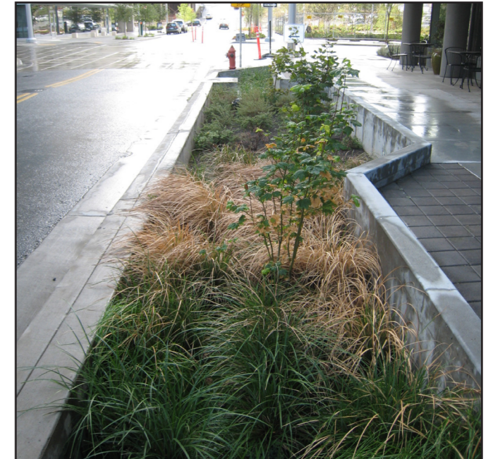
Stormwater tree pit with slotted curb, Portland, OR
