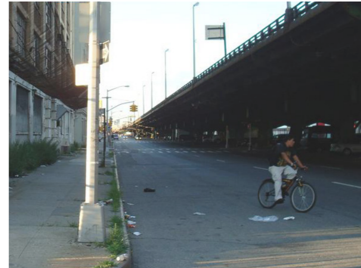
Third Avenue from 18th Street to 27th Street (existing)
