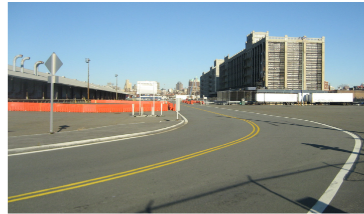
Pier 11 at Commercial Wharf (existing)
