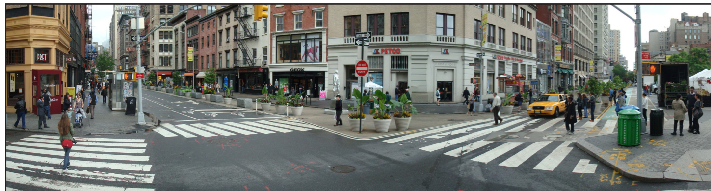
Sidewalk extension implemented in conjunction with high-visibility crosswalk striping, Union Square, Manhattan
