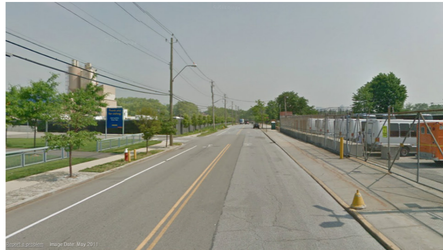
Columbia Street opposite Erie Basin Park (seen at left), view looking north (existing)
