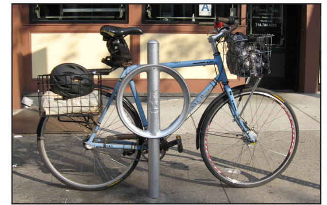
Standard NYC parking meter conversion to bike rack
