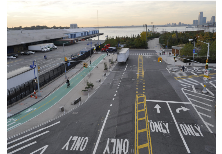
Recent improvements on Atlantic Avenue connection between Columbia Street Greenway and Pier 6
