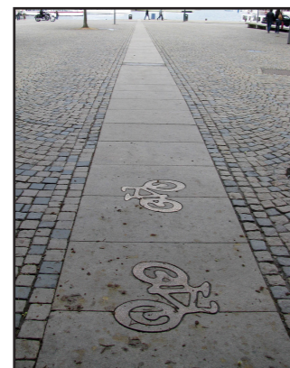
Belgium block street with stone slabs for cyclists with metal bicycle logo inlaid, Stockholm
