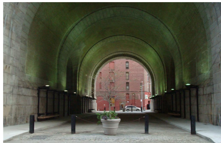
Water Street going under the Manhattan Bridge (existing)
