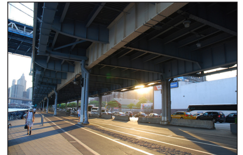
Manhattan Waterfront Greenway underneath the FDR Drive South, Manhattan
