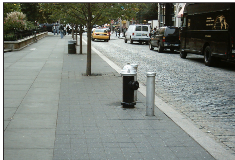
Decorative pavement materials (bluestone paving and square asphalt pavers on the sidewalk, extra wide granite curb and granite block in the road bed), Union Square West, Manhattan
