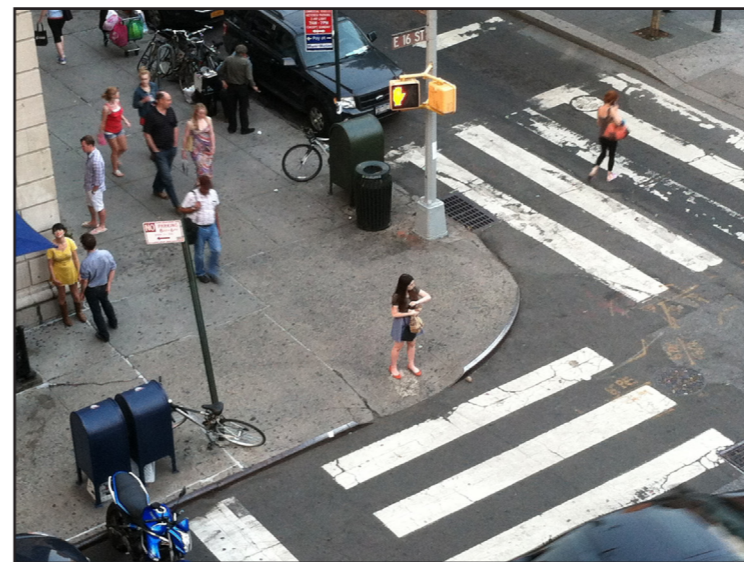
Street corner with reduced curb radius, Union Square West, Manhattan
