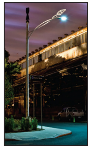
Day and night shots of the wind/solar powered street lights installed recently at the Brooklyn Navy Yard
