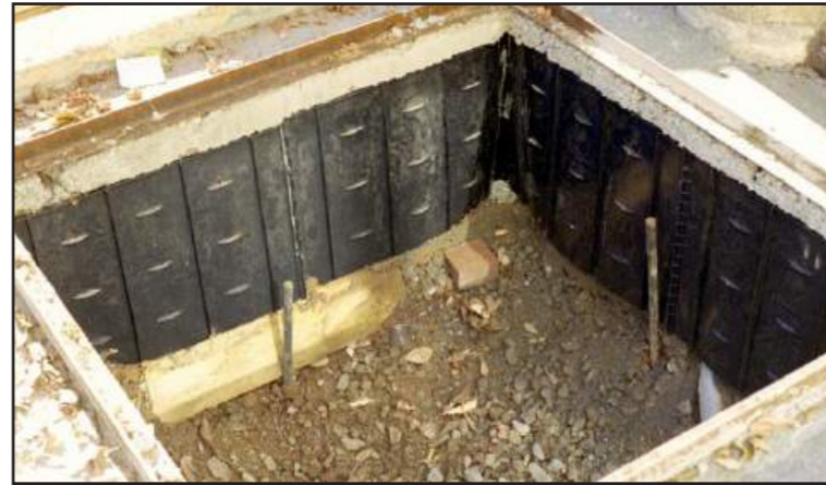
Root barriers prevent the roots from lifting the sidewalk but curtail growth
