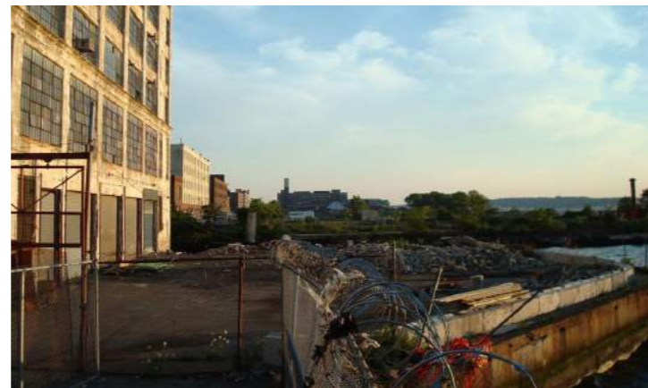
Marginal Street facing south from 39th Street (existing)
