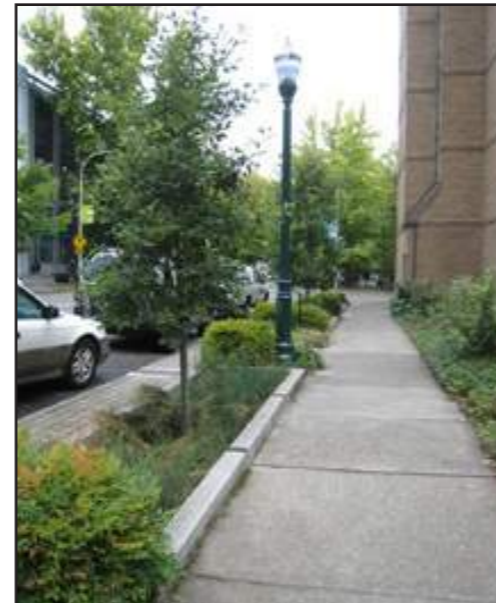
Slotted curb rain garden, Portland, OR
