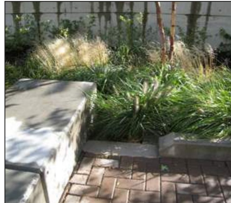
Slotted curb allows stormwater capture, Portland, OR
