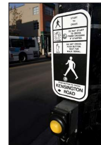
Pedestrian actuated signal, Calgary, Canada, Photo: PBIC
