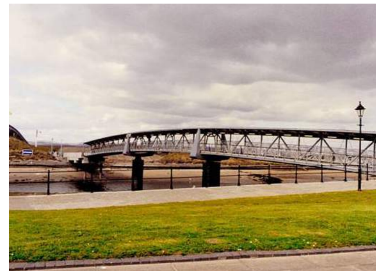
Small-scale operable pedestrian bridge; closed and open, UK (precedent)
