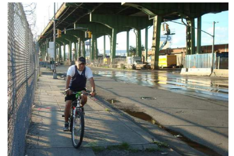
Hamilton Avenue at 17th Street facing west (existing)
