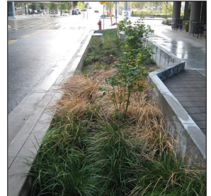
Stormwater tree pit with slotted curb, Portland, OR
