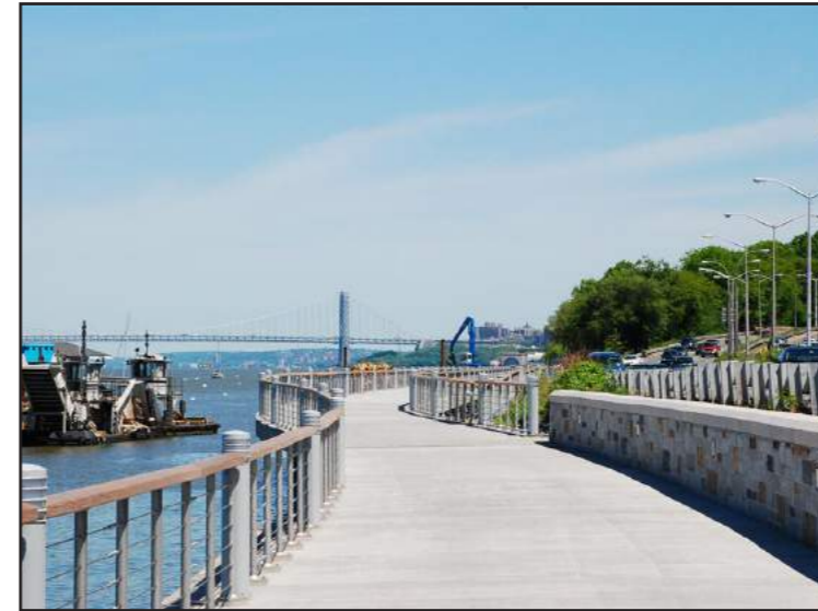
Multi-use path connection built on a pile-supported structure over the open water in Riverside Park, Manhattan
