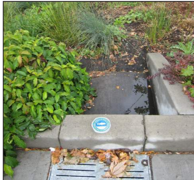
Storm drain outfall to rain garden, Portland, OR
