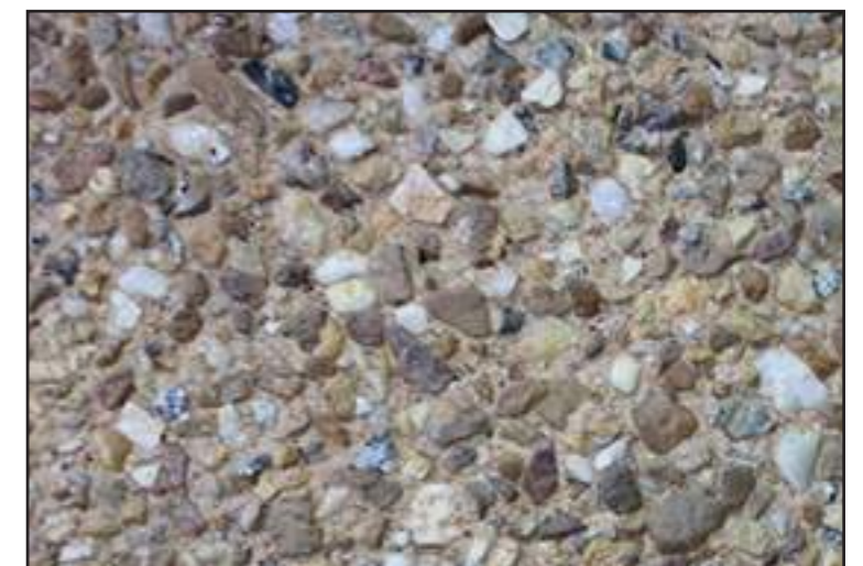
Detail of exposed aggregate concrete pavement
