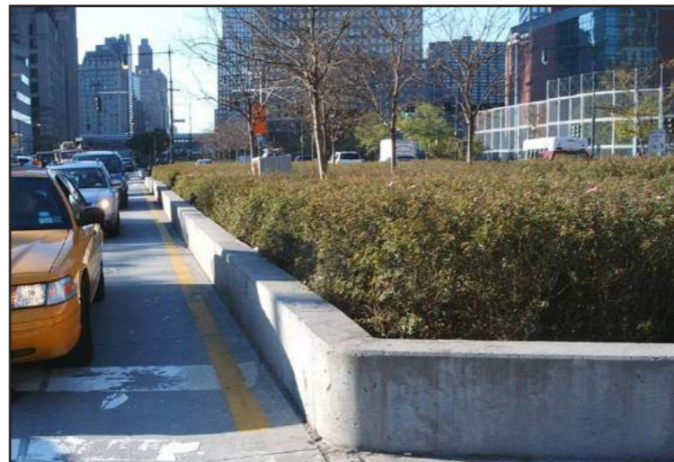
Planted roadway medians, Route 9A, Manhattan
