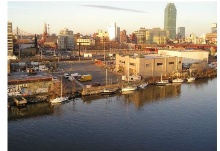
Newtown Creek facing north towards Queens (existing)
