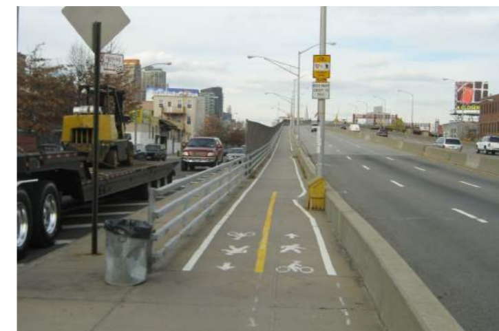
Pedestrian and bicycle path on west side of Pulaski Bridge (existing)
