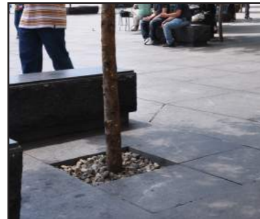
Paver grate suspension system with pavers installed, Battery Place, Manhattan
