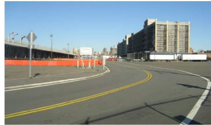
Pier 11 at Commercial Wharf (existing)
