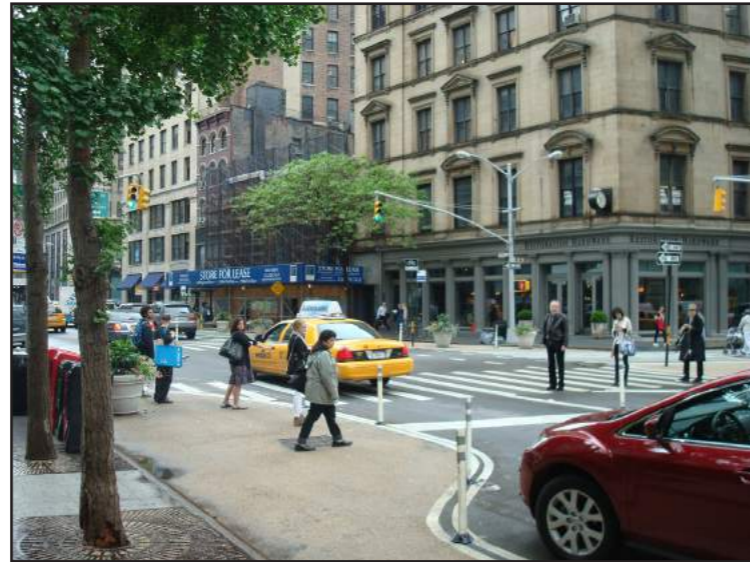
Curb extension implemented in epoxy gravel with flexible bollards, Manhattan
