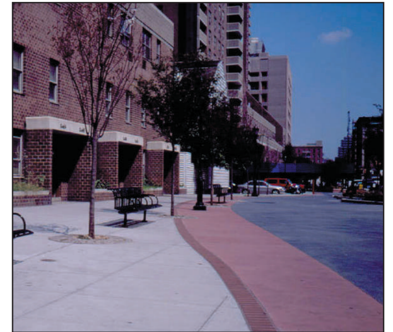
Red, white and gray colored concrete pavement on widened sidewalk on Greenwich Street, Manhattan
