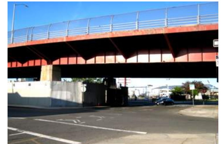
Box Street at the Pulaski Bridge (existing)
