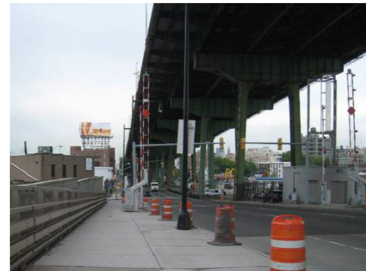
Hamilton Avenue Bridge looking west (existing)
