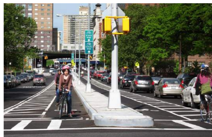
Grade-separated bicycle lane on Sand Street (existing)
