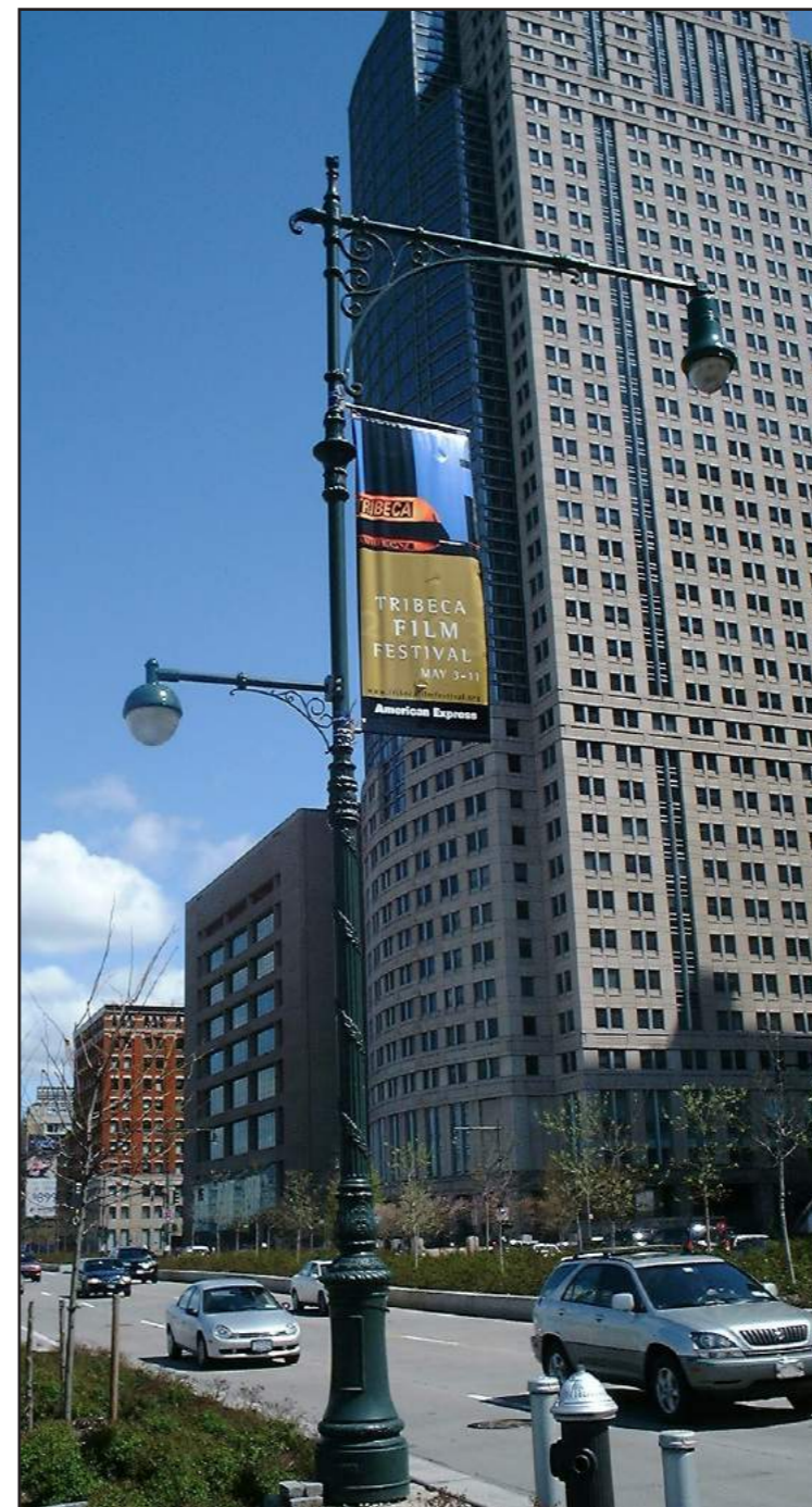
NYCDOT typical historic Type M with pedestrian-scale light head, Route 9A Bikeway, Manhattan
