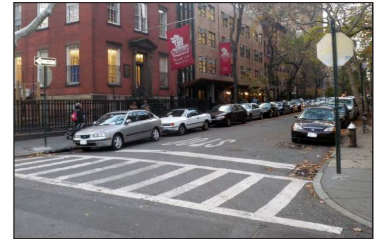
NYCDOT school safety (ladder style) crosswalk—used only along designated walk to school routes, Manhattan
