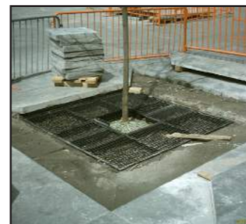
Paver grate suspension system without pavers installed, Battery Place, Manhattan
