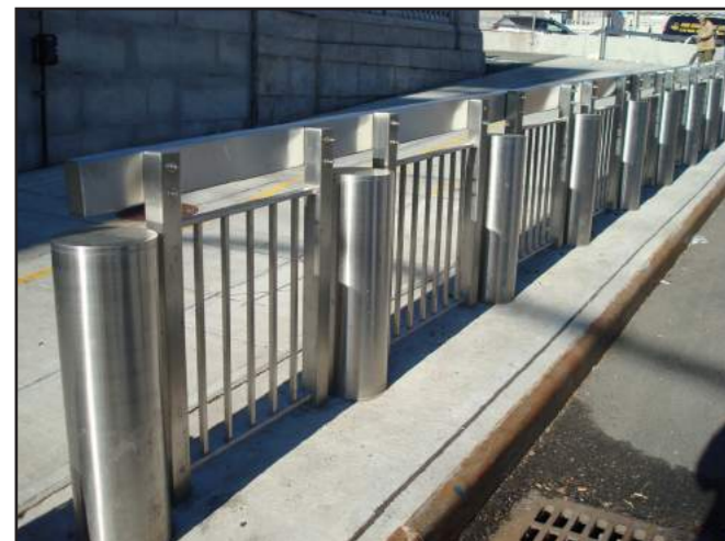
Combination bollard and railing, Manhattan Bridge Approach, Manhattan
