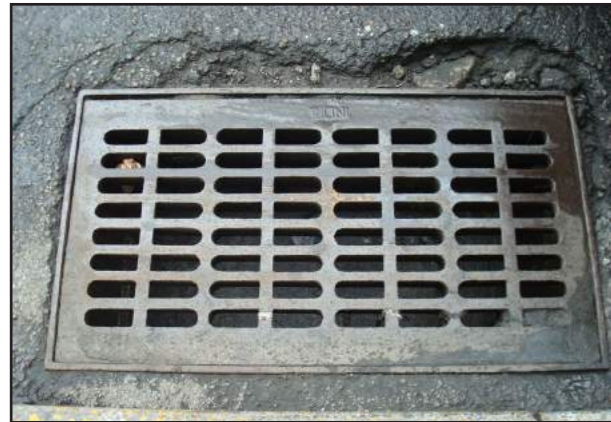
Bicycle-safe drainage grate
