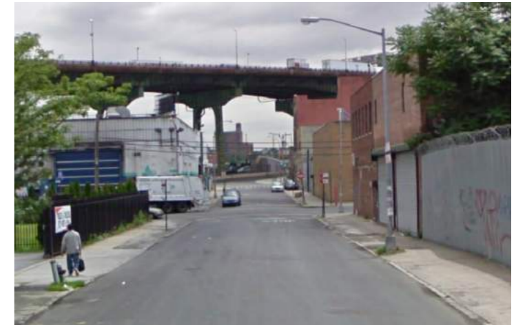
Lorraine Street between Clinton and Court Streets looking east (existing)
