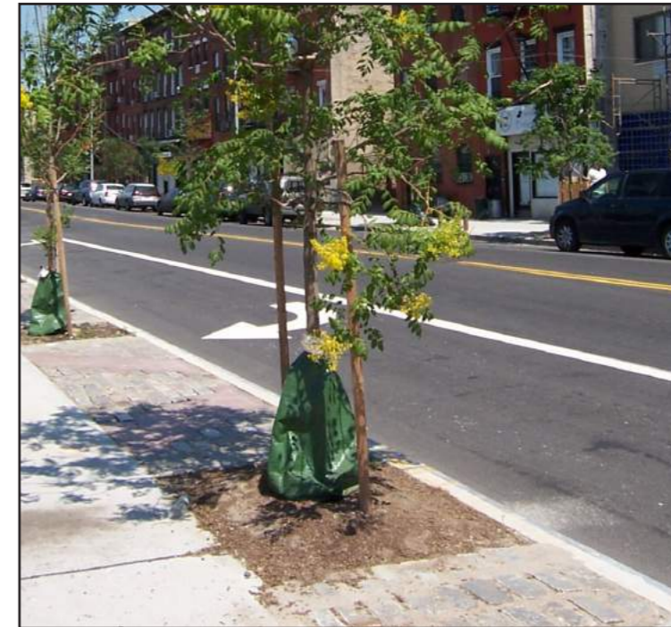
Cobblestone pavement with porous sand joints, Columbia Street, Brooklyn
