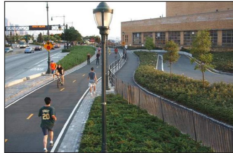
Off-street multi-use pathway with separation between bikes and pedestrians, Route 9A Bikeway/Walkway, Manhattan
