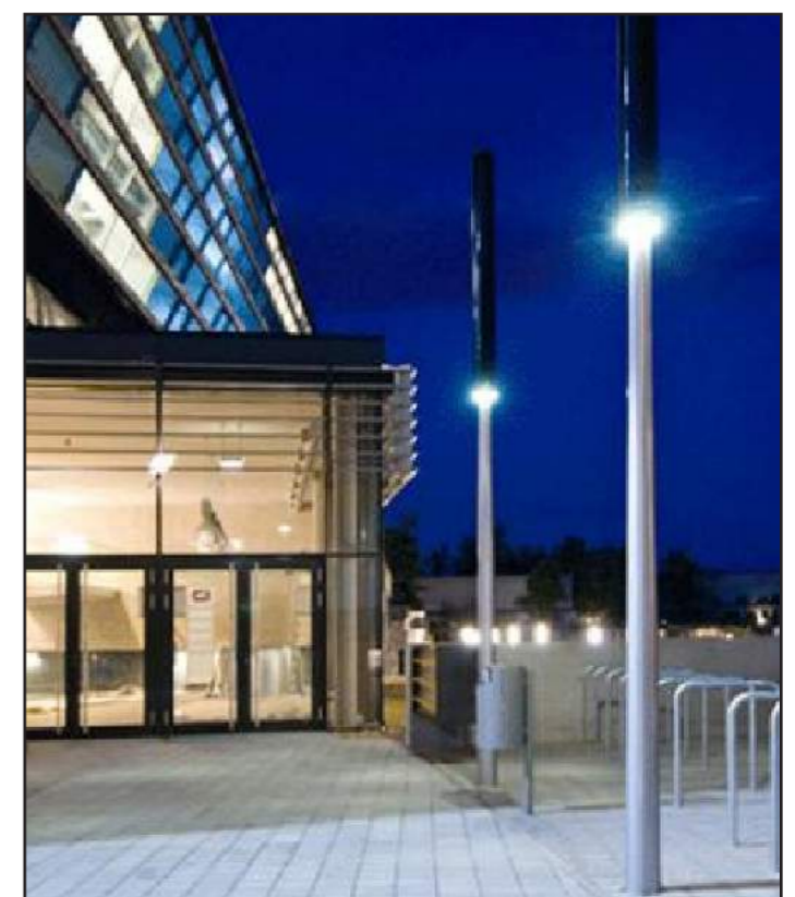
Solar powered LED plaza lighting, Spain
