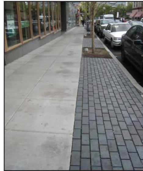
Porous pavers in amenity strip
