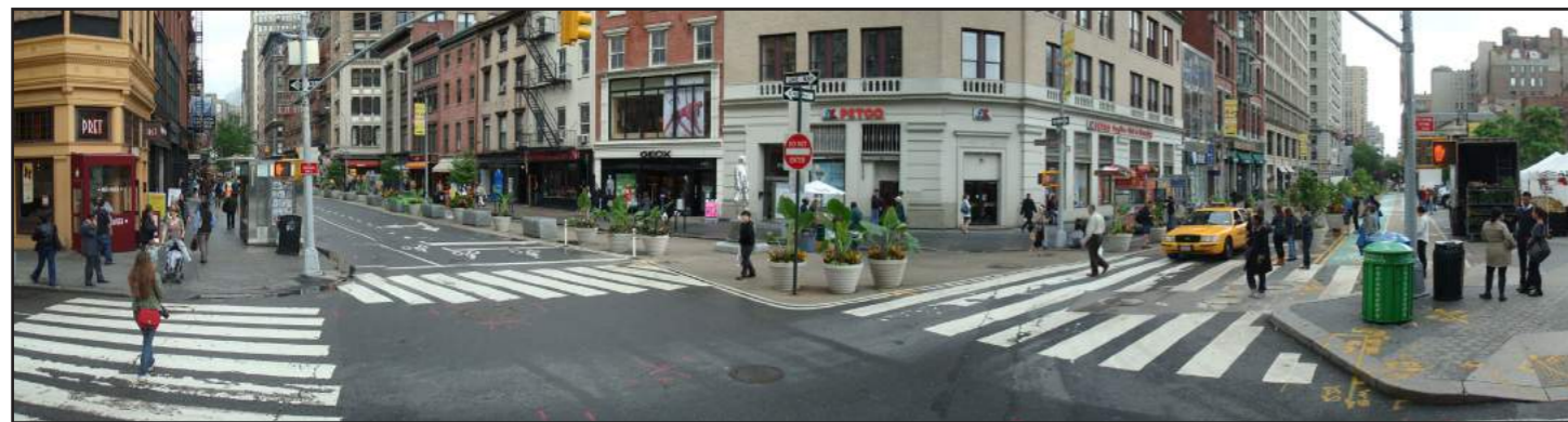
Sidewalk extension implemented in conjunction with high-visibility crosswalk striping, Union Square, Manhattan
