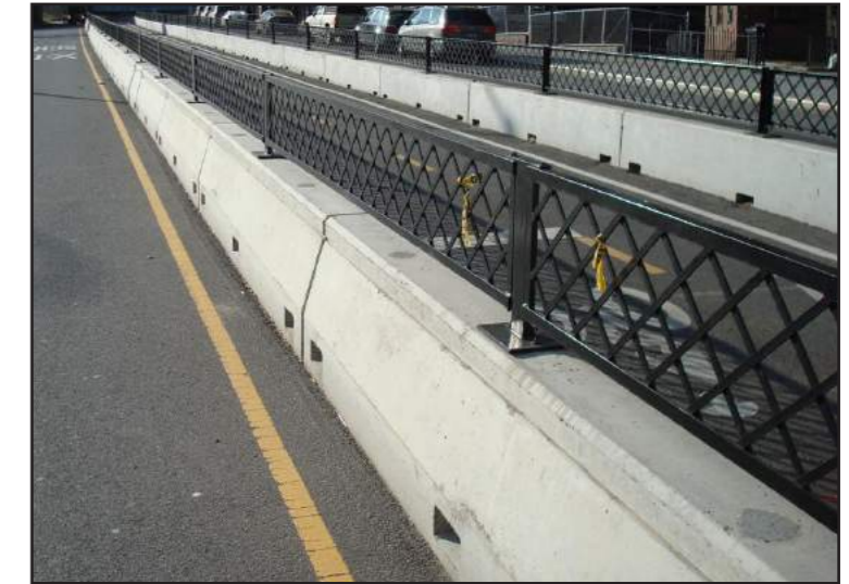
Reinforced concrete divider with railing, Sands Street, Brooklyn
