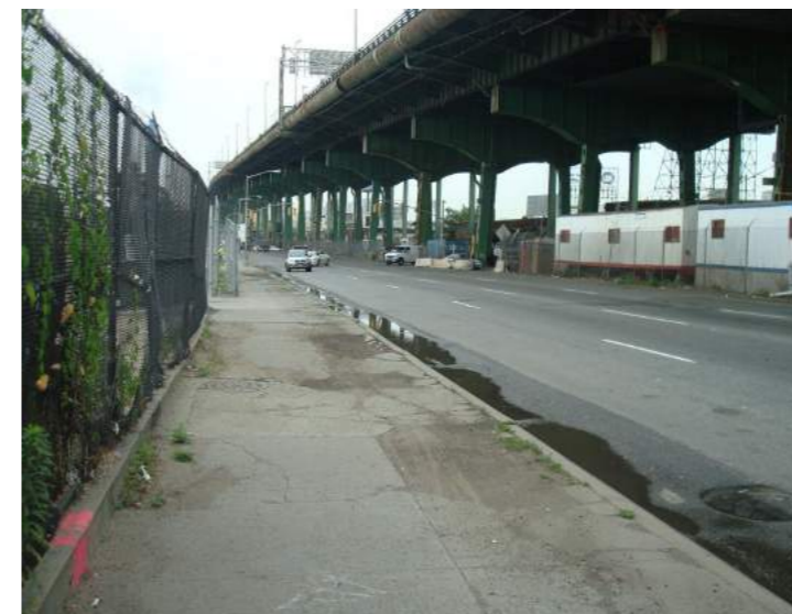
Hamilton Avenue looking west from Department of Sanitation Marine Transfer Station (existing)
