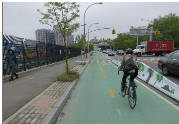
Jersey barrier separated two-way path, Columbia Street, Brooklyn
