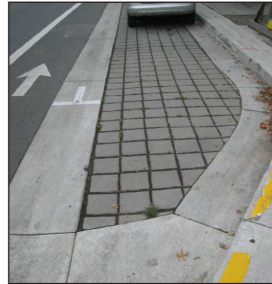
Porous pavers in parking lane
