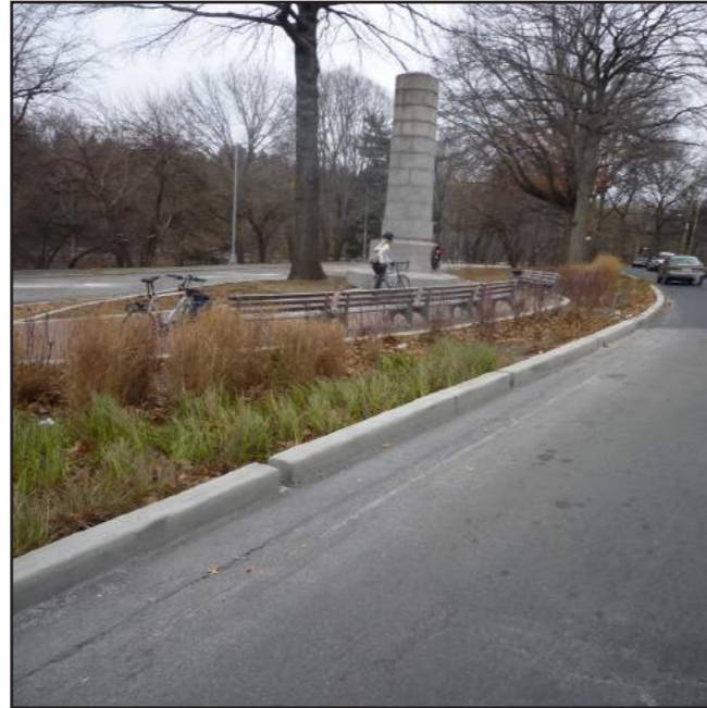
Slotted curb for natural percolation, Bronx River Greenway
