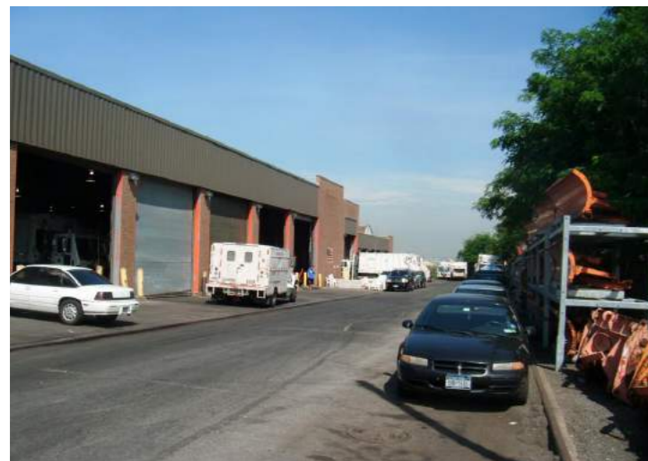
51st Street facing west from First Avenue (existing)
