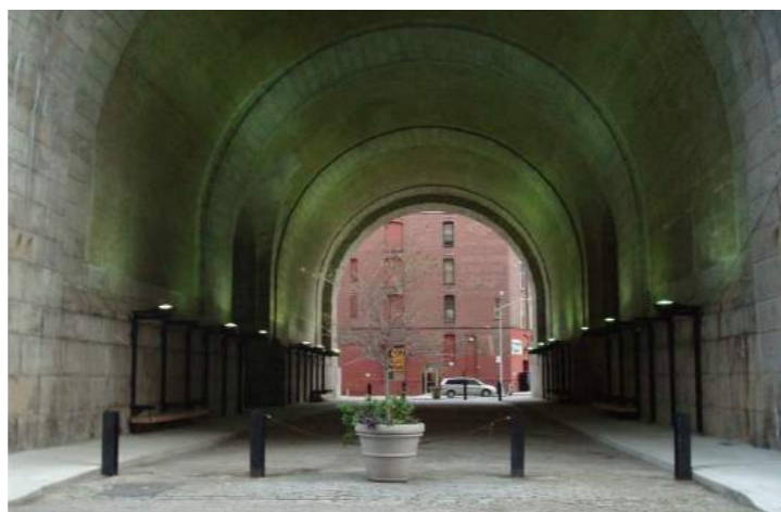
Water Street going under the Manhattan Bridge (existing)
