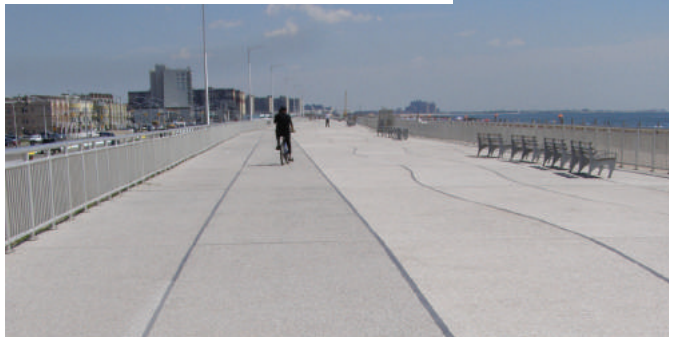
Reconstructed Rockaway Boardwalk path
