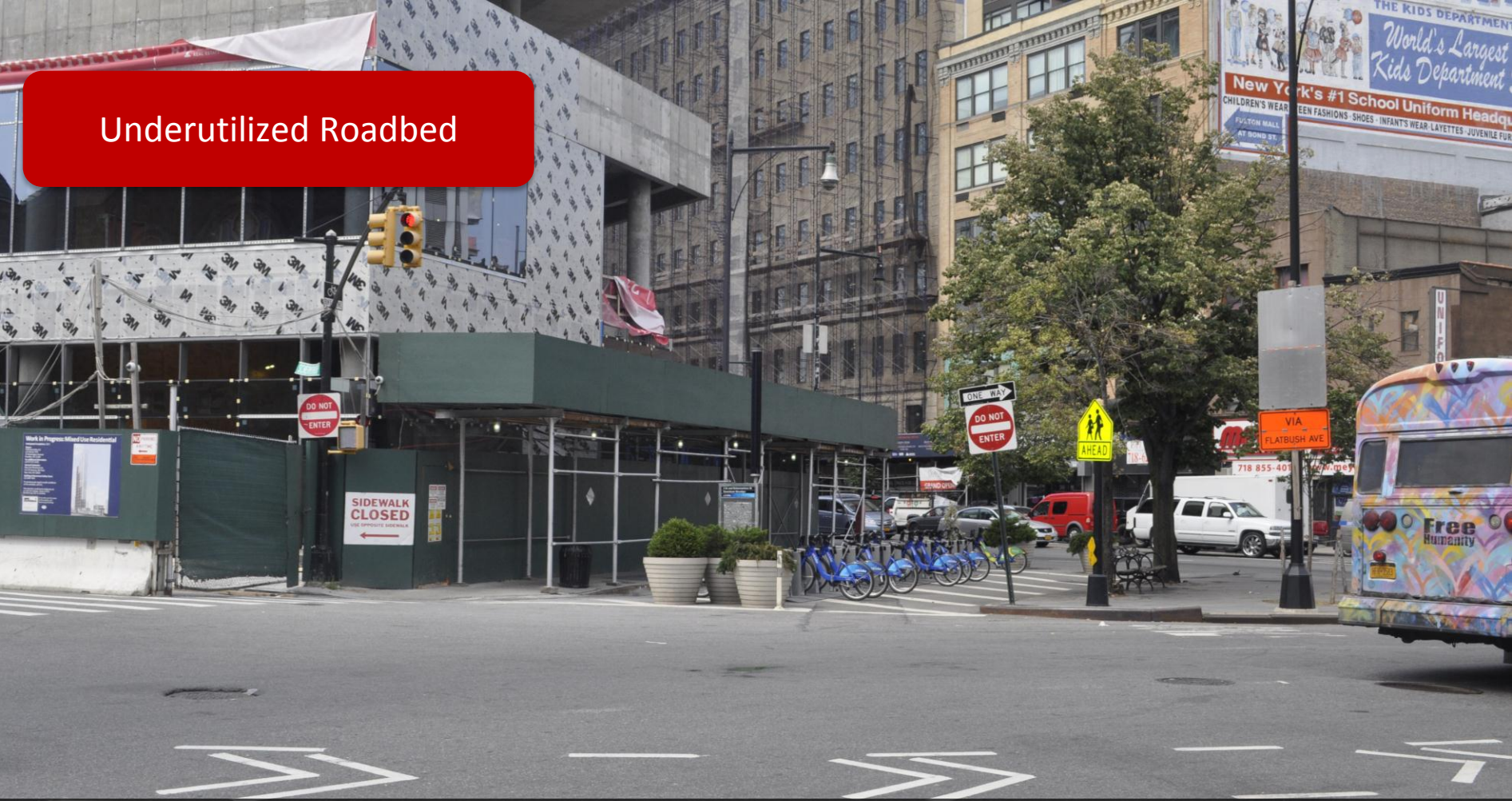
3rd Avenue Slip Lane @ Schermerhon St (looking north)
