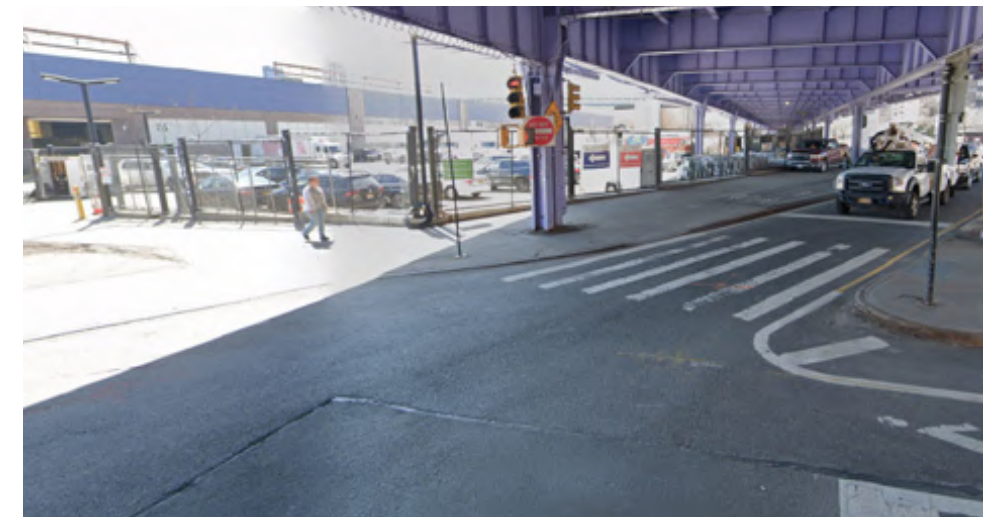
Montgomery Street Crossing under FDR viaduct
