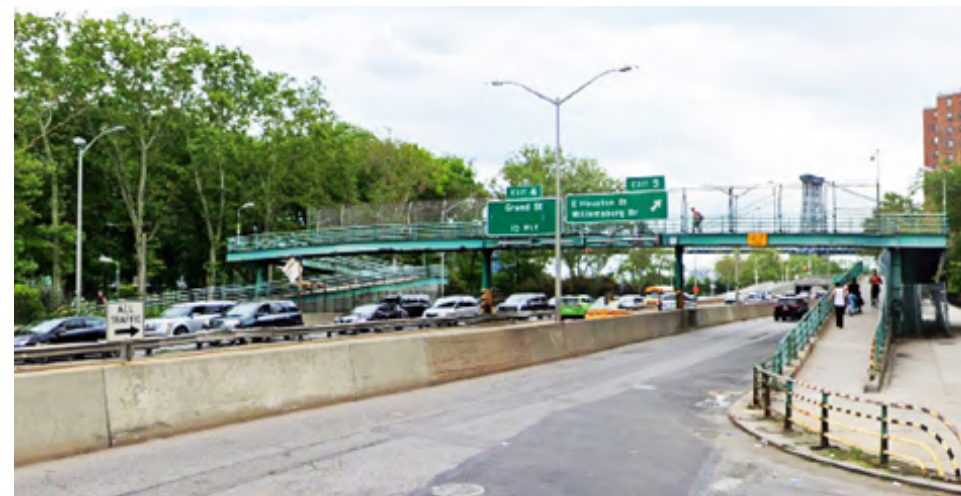
East 6th Street bridge city-side landing.
