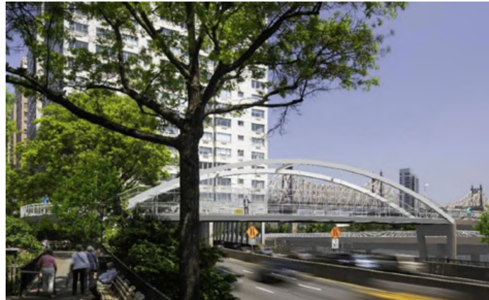
East 54th Street Pedestrian Bridge, Manhattan
