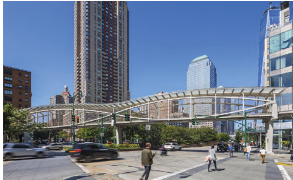
Robert R. Douglass Bridge, Manhattan
