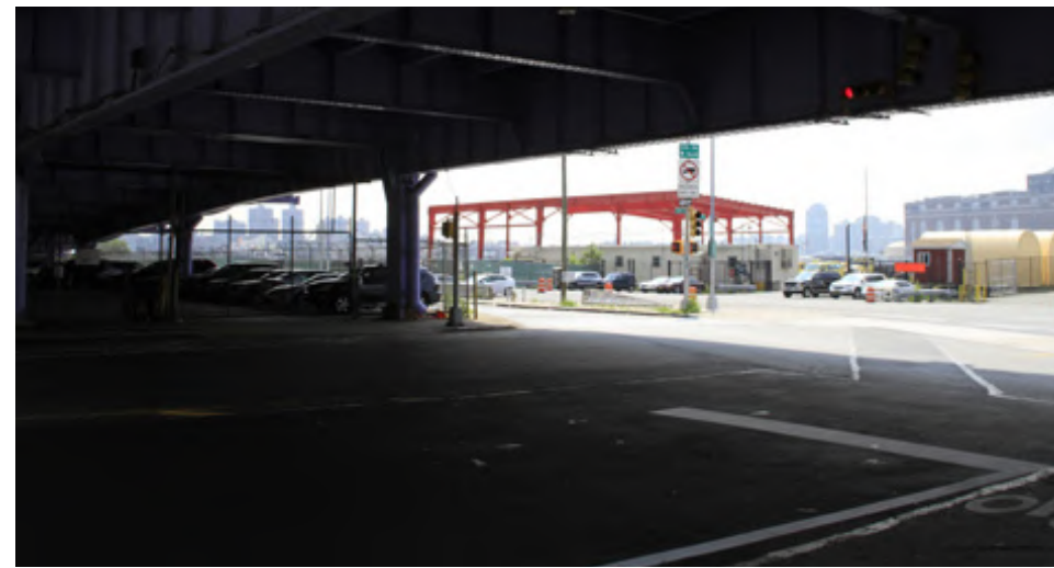
Montgomery Street and FDR on ramp
