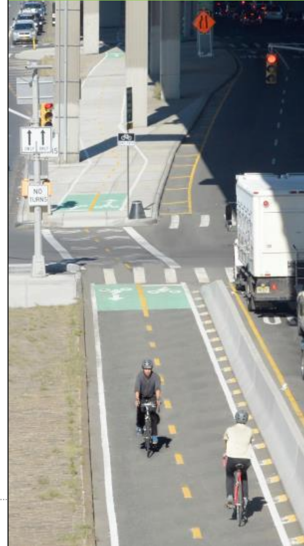
Under Elevated Structure Protected Lane
