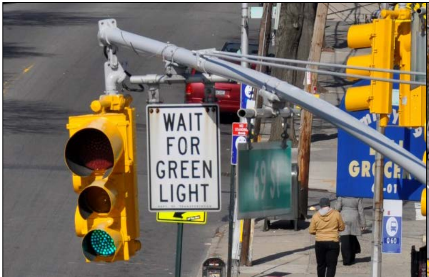
New signal construction
