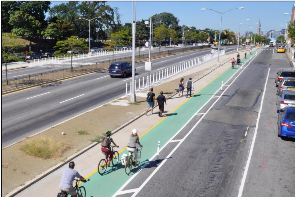
Pedestrian path, bike lane, and slip closure
