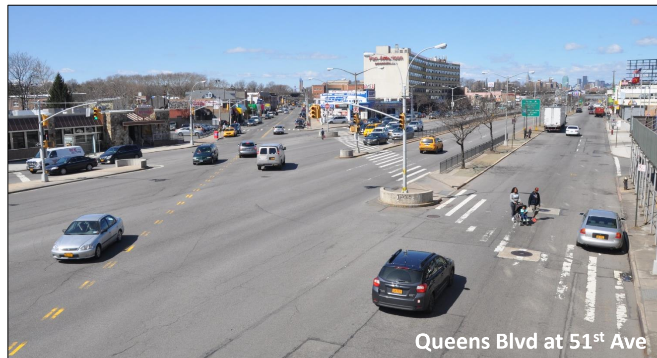
Wide road / Long crossing distances
