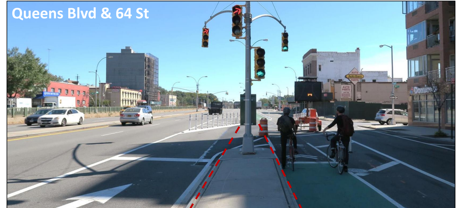
New slip lane between mainline and service road
