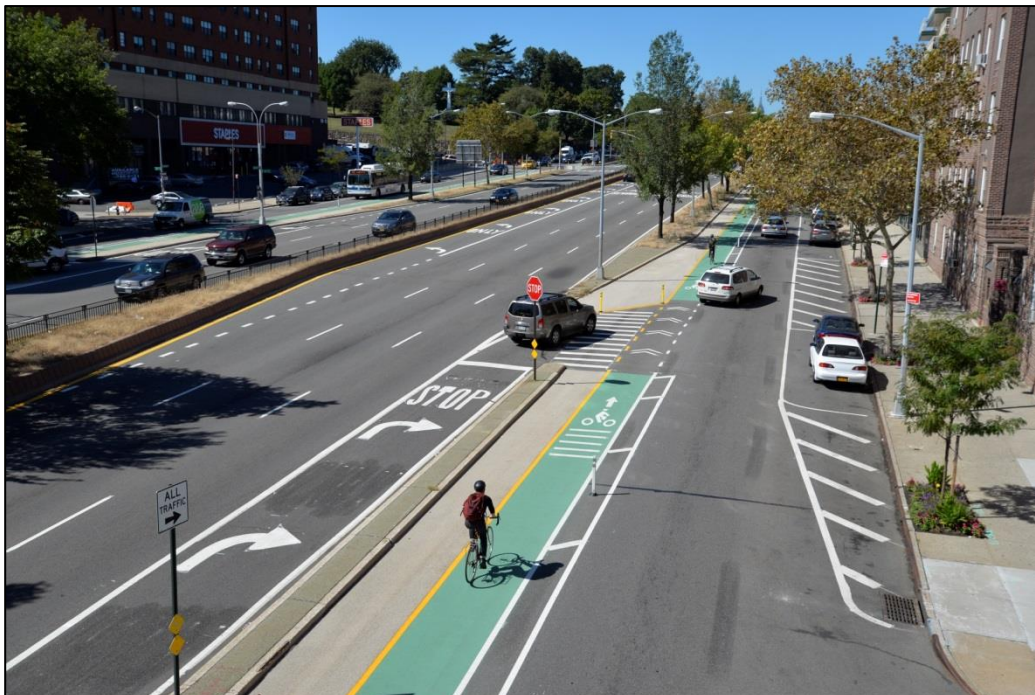
Stop controlled slip lane
