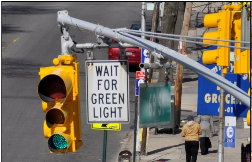
New signal construction
