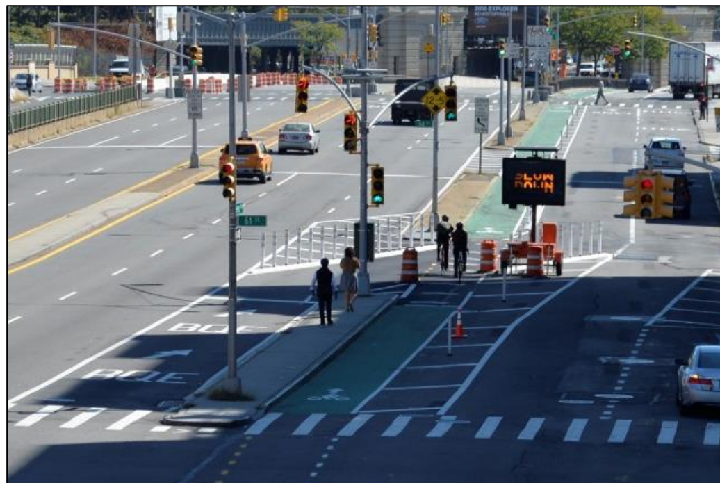
Slip lane with new traffic signal
