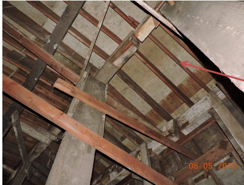
Underdeck looking upwards
