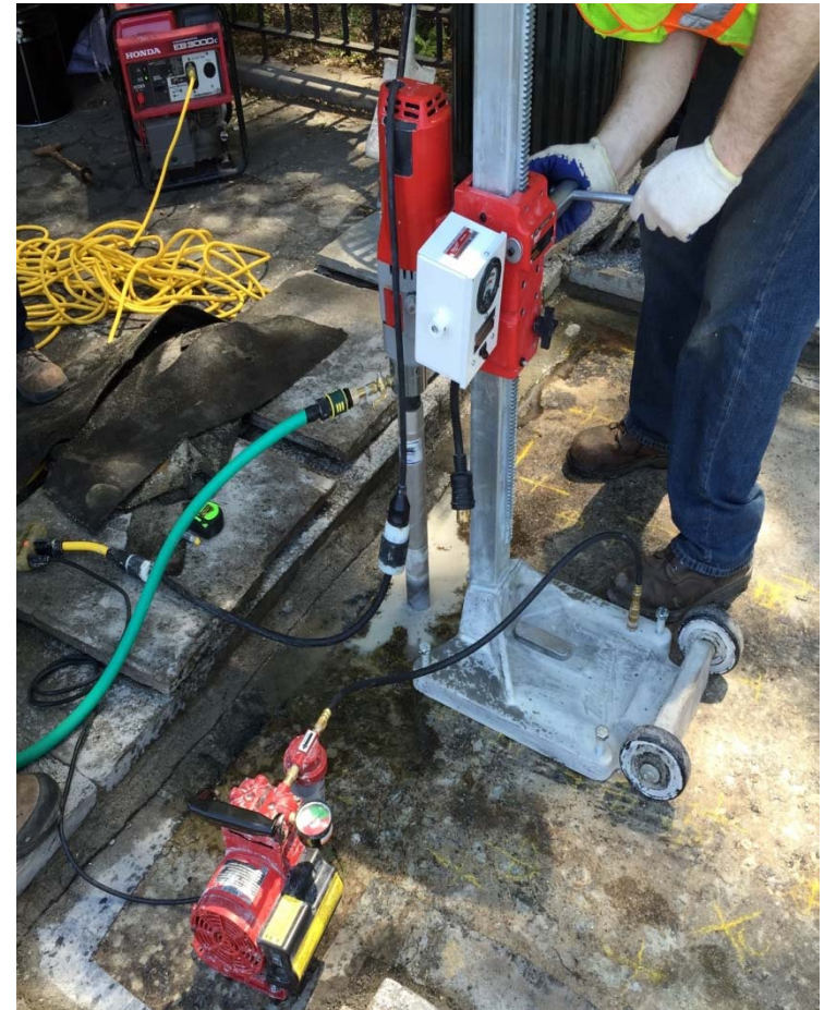
Concrete coring
