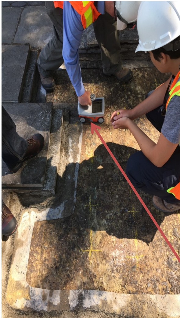
Ground Penetrating Radar to locate rebars
