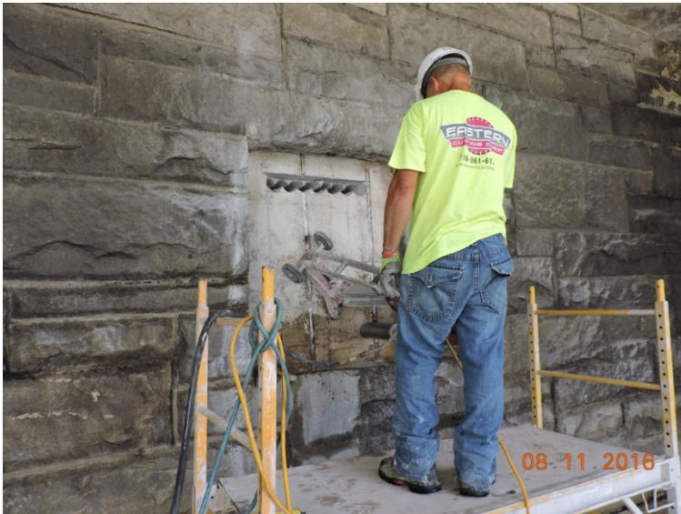
Removing concrete for access
