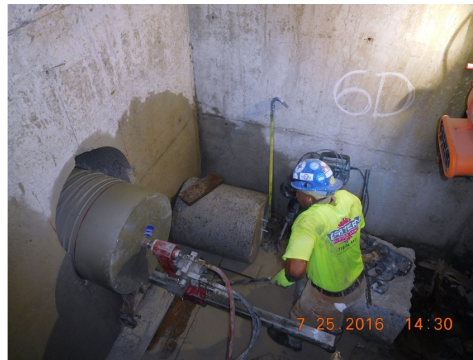
Transverse Access being created
