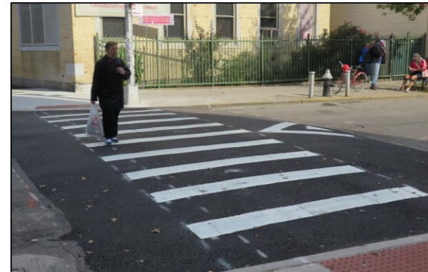
Raised crosswalks/intersections: allows for pedestrians to cross at grade and reduces vehicle speeding
