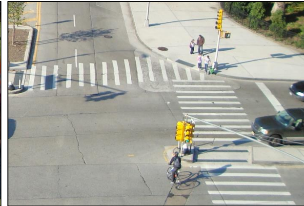
Close slips/normalize turns: creates safer turns and improves driver to pedestrian visibility
