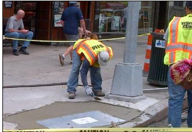
Repair pedestrian ramps: repair pedestrian ramps on intersections with safety projects
