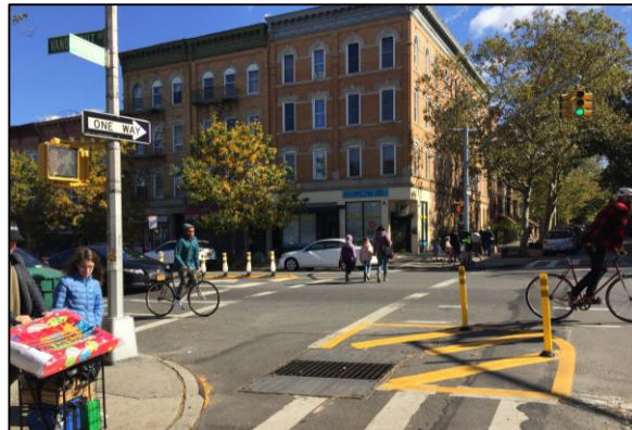
Left Turn Traffic Calming: Modifies turning angle from cross street to create safer, slower left turn
